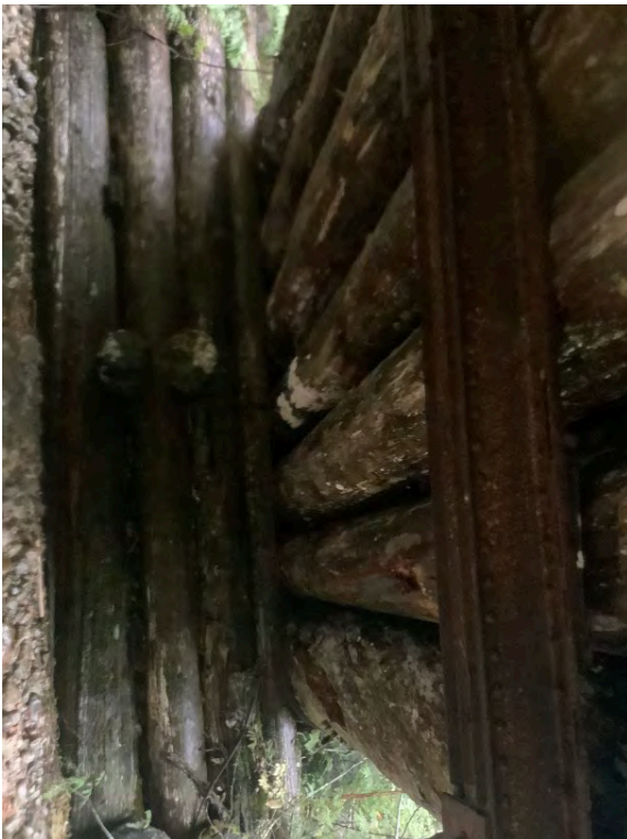
Left Bank Abutment when facing downstream
